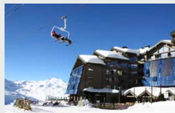
HOTEL ALTAPURA Architect: Studio Arch, Tresserve Client: Hôtel Altapura, Val Thorens Fabricator: Serag Aluminium, Montbonnot-Saint-Martin Reynaers system: CW 60 Solar
